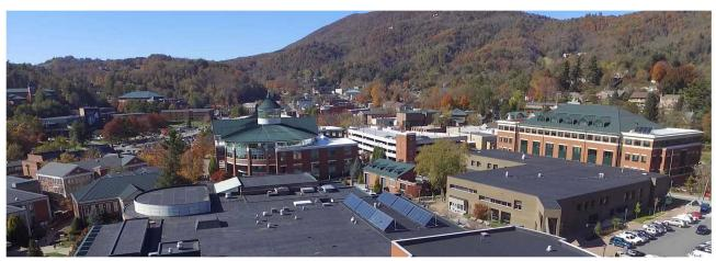
The 35-panel Plemmons Student Union solar-thermal system, pictured in foreground, was the first large-scale system installed on campus in 2009. This system preheats water used in restrooms, fitness center locker rooms and the building's food service areas. The most recent solar-thermal system installed on campus, pictured on the right, is located on the Reich College of Education (RCOE). This system uses four panels for preheating water for RCOE restrooms.
