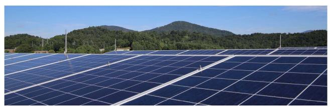
The PV system on the roof of Leon Levine Hall is comprised of 214 panels, with 57.8kW of capacity.
